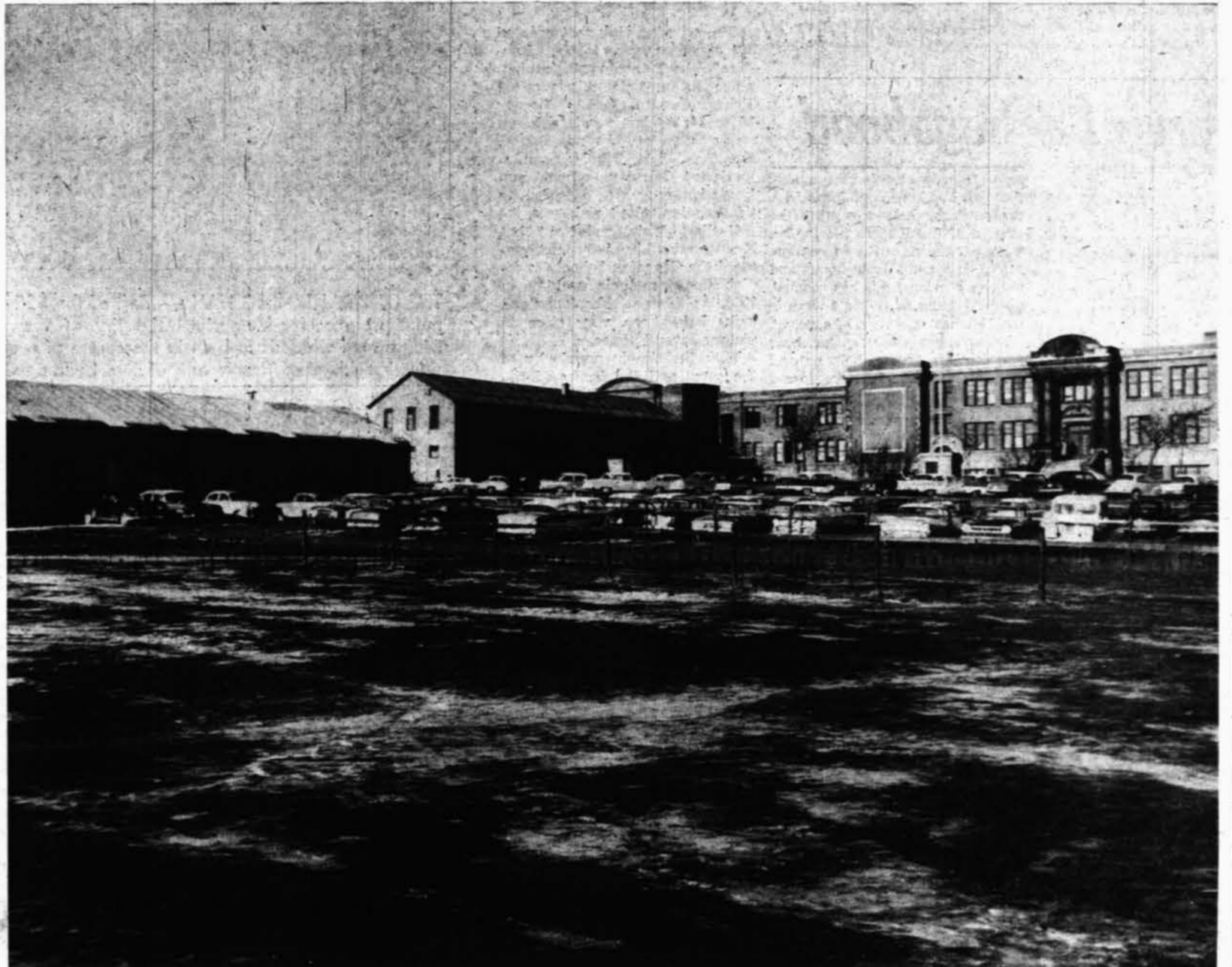
MEMORIAL UNIVERSITY — Quonset huts and temporary buildings comprise a large part of the current Memorial University of Newfoundland shown in the above photograph. The one and only permanent structure seen on the right hand side of the picture used
