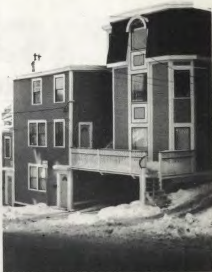
Long's Hill Apartments
