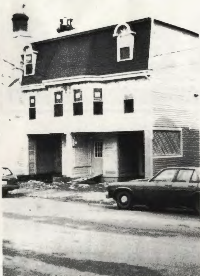
Infill housing under construction on Queen's Road near Rawlin's Cross.
